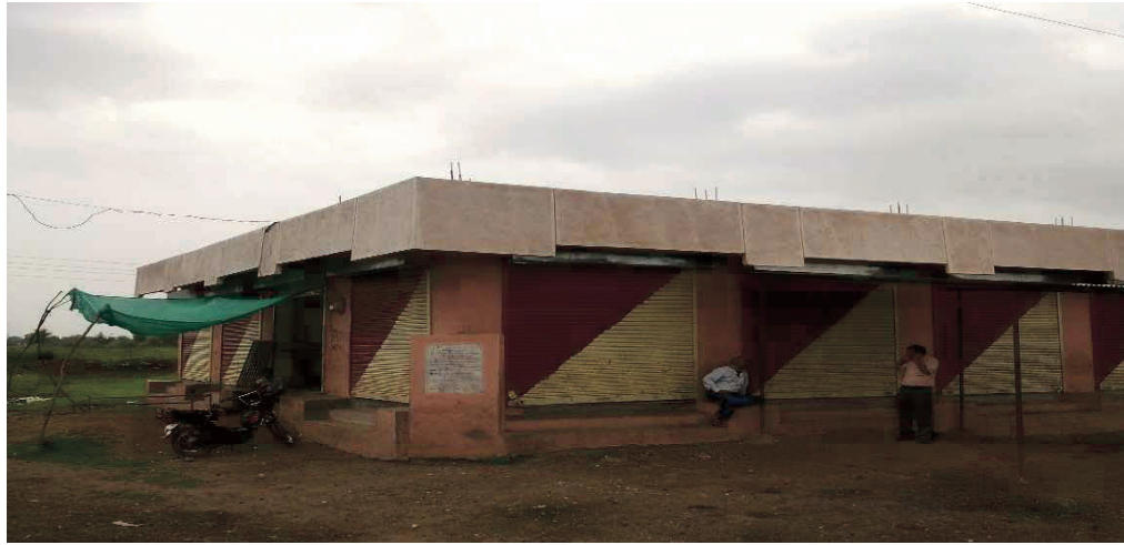
Commercial complex constructed instead of community hall at Nimkarda, Taluka- Balapur, district Akola
